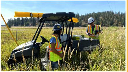
Now through November, you may see PUD contractors testing our wood poles to maintain system reliability. Crews will have PUD signage, wear safety gear, and carry ID. They may use ATVs and will knock before entering private property. The process includes drilling to test pole integrity, tagging, and documenting poles. For questions, please contact us.
