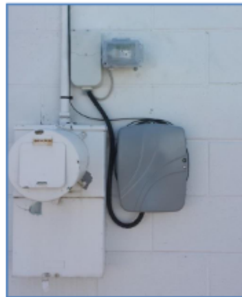
(Example of CPE installation)
